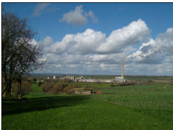
(b) One of the most dominant landmarks in the district – the cement factory
