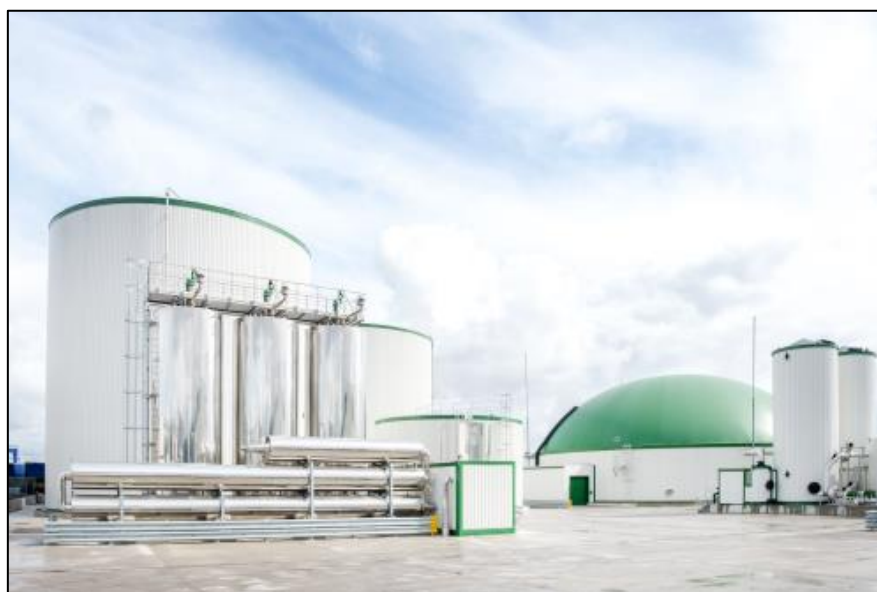
Figure 3: Refood Anaerobic Digestion facility, Widnes
