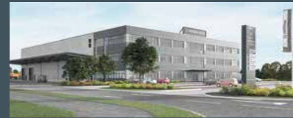
UK: New building for the Winthorpe subsidiary. Completion scheduled for summer 2018.
