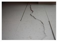
FIGURE 7. A FLOOR SLAB OVER PYRITIC SHALE FILL AND DOWELED INTO A PERIMETER GRADE BEAM EXHIBITED A LARGE CRACK WITH VERTICAL OFFSET AND ROTATION ABOUT THE DOWEL POINT INTO THE GRADE BEAM.
