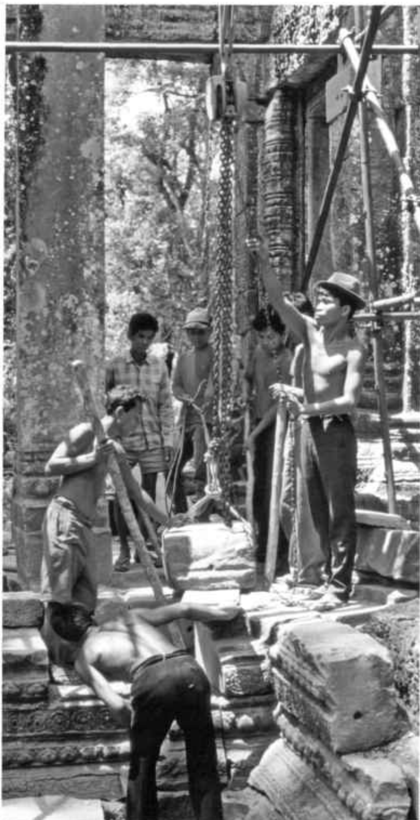
WORKERS STABILIZE ONE OF THE TOWER ENTRANCES TO ANGKOR'S PREAH KHAN
