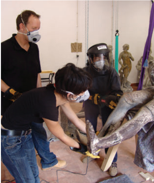
Figure 5. Cutting Autumn to remove the old, corroded iron structure.
