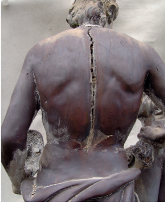
Figure 7. Crack in the back of Vertumnus , caused by expansion of internal iron armature.
