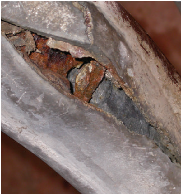
Figure 3. Fissure in Autumn 's leg, through which it is possible to see the severe corrosion of the iron inner structure.
