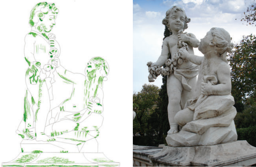
Figure 2. Putti. Left: Condition survey mapping prior to the biocide application (September 2006). Right: General appearance after two years of the biocide application (October 2006).
