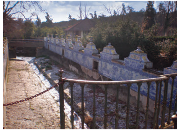
Figure 3b. End of the decorated structure adapted from an early-twentieth-century conservatory. Below the bridge, at the end of the canal, the flood gate was installed. Note that the azulejo decoration is over one meter from the floor.
