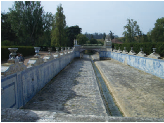
Figure 3a. The beginning of the Canal de Azulejos proper. In the distance, the center block. Note that the azulejo cover starts right at the floor of the canal and, as this slopes down, the undecorated wall becomes evident as can be seen in the center block.
