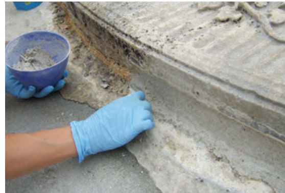
Figure 9. Sealing joints in one of the Shell fountains.
