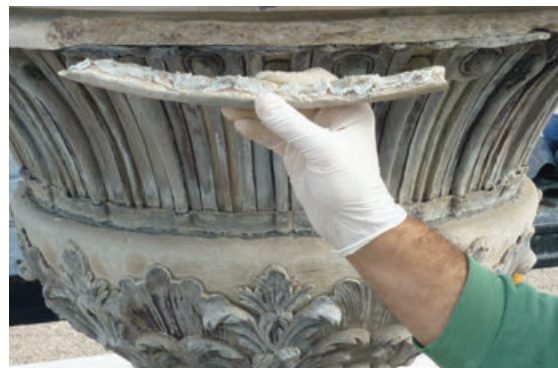
Figure 11. Reattaching a fragment of the Lioz limestone vase of one of the Monkey fountains.
