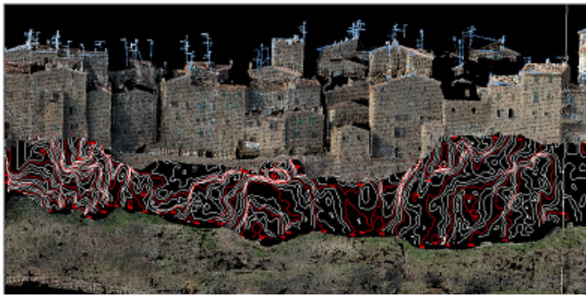
Figure 3 – Example of spot elevation of the cliff obtained from the laser scanner survey
