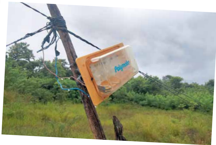
New, more durable light covers than the previously used shower heads have been introduced and will be helpful in reducing fence maintenance cost significantly © Supun Lahiru Prakash
