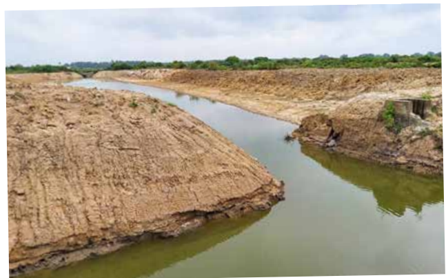
Newly dredged canals
