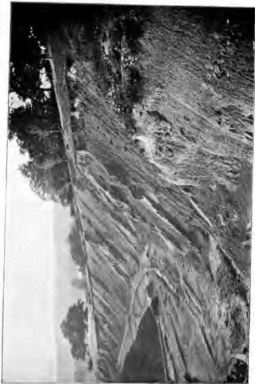
THE TEMESIDE AND BOTTOM-BEDS OF THE OLD RED SANDSTONE IN THE APPROACH-CUTTING TO THE LEDBURY TUNNEL.
