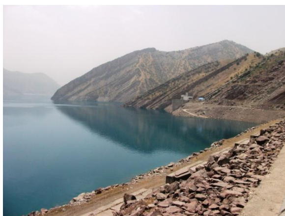
Figure 8-14: Nurek reservoir from dam crest
