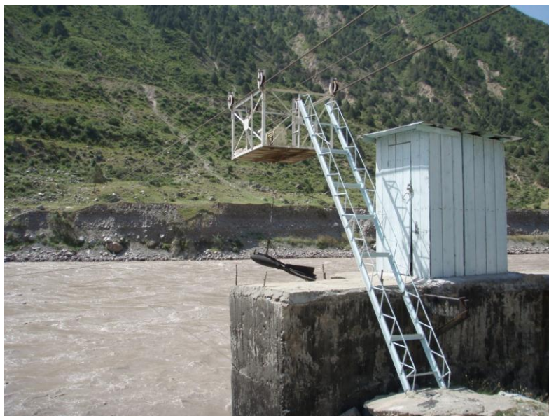
Figure 8-25: Darband hydrological station
