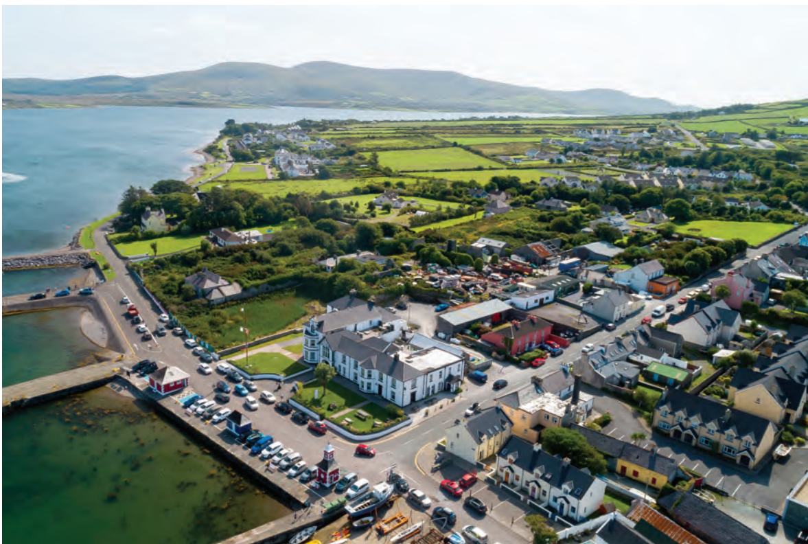
Figure 10 First Message Building and Slate Yard, Knightstown, Valentia Island, Co. Kerry. (Alan Landers).
