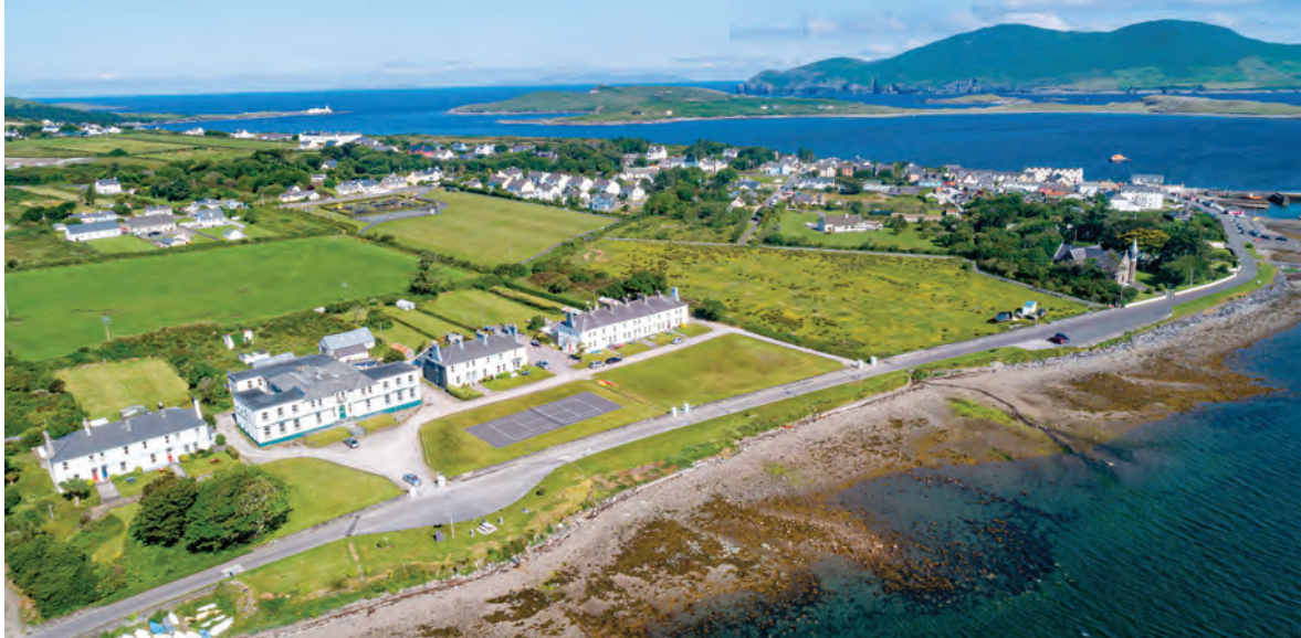
Figure 9 Valentia Cable Station and Cable Terraces, Knightstown, Valentia Island, Co. Kerry. (Alan Landers).
