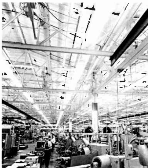
The inherent linear nature of fluorescent lamps suits them well for many industrial lighting applications. In this TRW Equipment plant in Euclid, Ohio, the lighting provides 100 to 125 footcandles at the working level.
