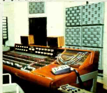
... extended low frequency response can be achieved simply by spacing panels away from walls...
