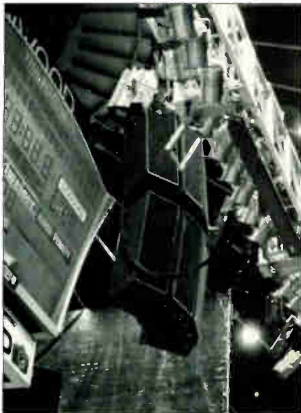
One of the four groups of eight MSL-3 loudspeaker enclosures, arrayed for 360-degree coverage.
