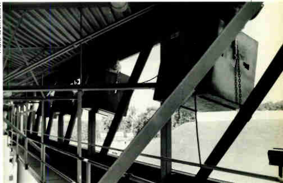
Sixteen OAP DP1810 boxes supplied by FBN Audio provide coverage for the lawn area at the Starwood Amphitheatre.
