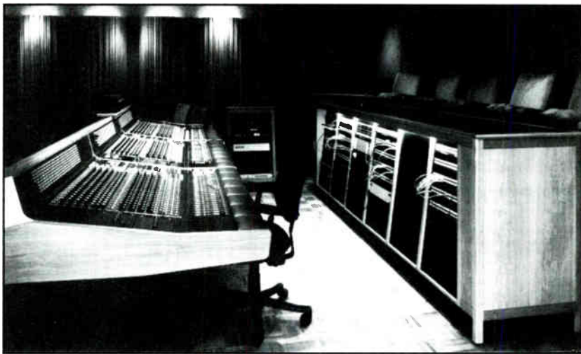
The Saul Zaentz Company Film Center - Stage 2 Installation
