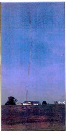
Fig. 1: The tower shows a serious bend.
