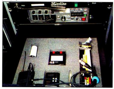
KIRO(AM)'s Marti RPU system features a 3dB gain omnidirectional screw-on replacement antenna (upper left, in drawer) and a Lectrosonics wireless transmitter (lower left).
