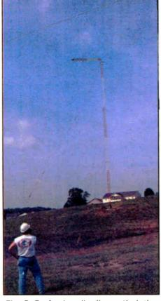
Fig. 2: Professionally dismantled, the tower is allowed to fall on itself.
