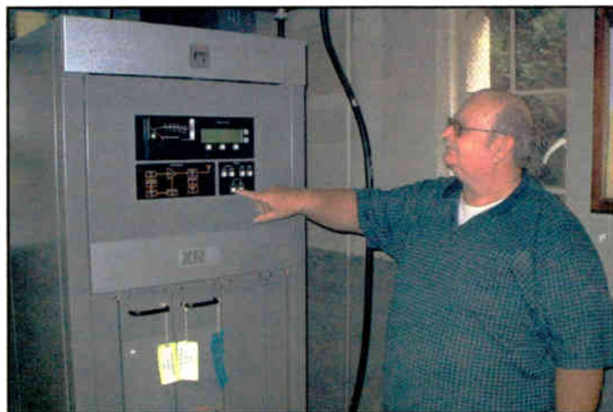
Bob Holcomb, Fisher Radio transmitter supervisor, with KVI's Nautel XR12, the first XR Series transmitter in that market.
