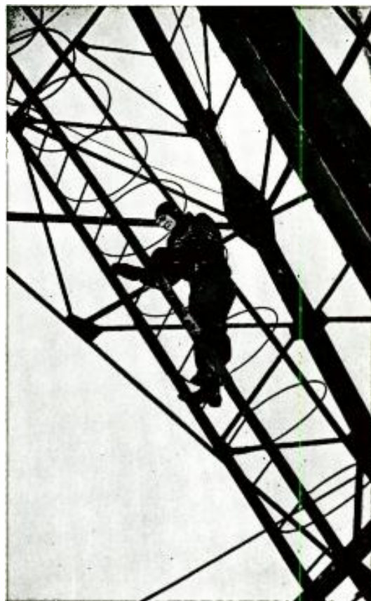
A Rigger descending the television mast at the BBC Television Station at Alexandra Palace, London. The mast, which rises to a height of 300 feet from the ground and stands on a hill 306 feet above sea level, carries vision and sound aerials on outriggers. (By courtesy BBC.)
