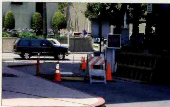
The transformer vault is accessed through this underground opening.
