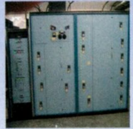
Kintronic Phasor Cabinet/ Control Rack Installed At KNWC-AM 5/2.3kW 1270kHz Five Tower DA-2
