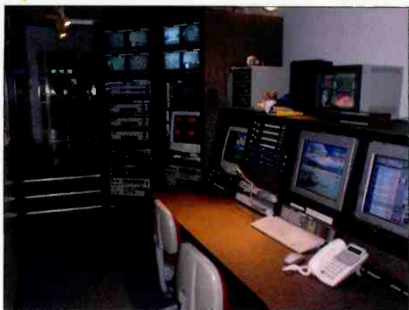
All feeds from KCSB-TV and ICTN go through master control before leaving the building. A BlueLine Automation Suite is central to the multichannel master-control operation and communicates with BlueLine video servers to ingest and recall on-air programming. Two master control racks next to the console are home to monitors and tape machines for recording and duplication.
