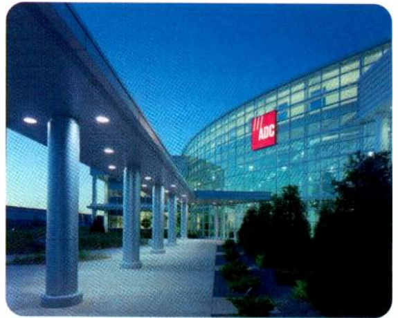
ADC's state-of-the-art facility in Shakopee, MN
