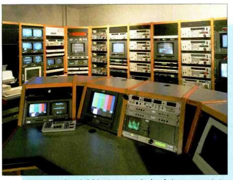
Master control console. L-R logo inserter control and marginoing, network monitoring, router control and logging computer display.
