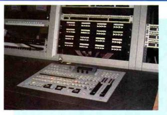
The central component of tae new facility is the Sony serial digital master control switcaer.
