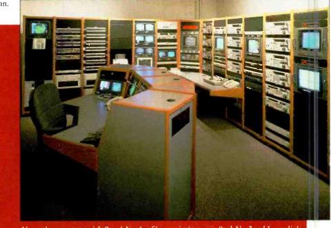
Network mas er corneo. L-P. rack No. 1--- fiber receive/mansmit. Rack No. 2 and 3--- audio/ video patching. Rack No. 4 --- character generation and control. Rack No. 5 --- network monitoring. Rack No. 6 'corner)--- er gineering station and monitoring. Rack No. 7--- network record and playback. Racks No. 8-12--- commercial insertion.
