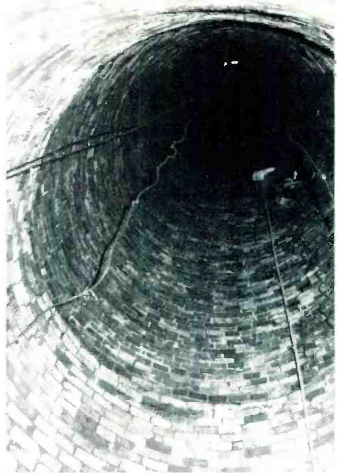
While rigging the (tapered) chimney for hoisting heliax, riggers have to climb what feels like the wrong side of a ladder 165 feet, in the dark
