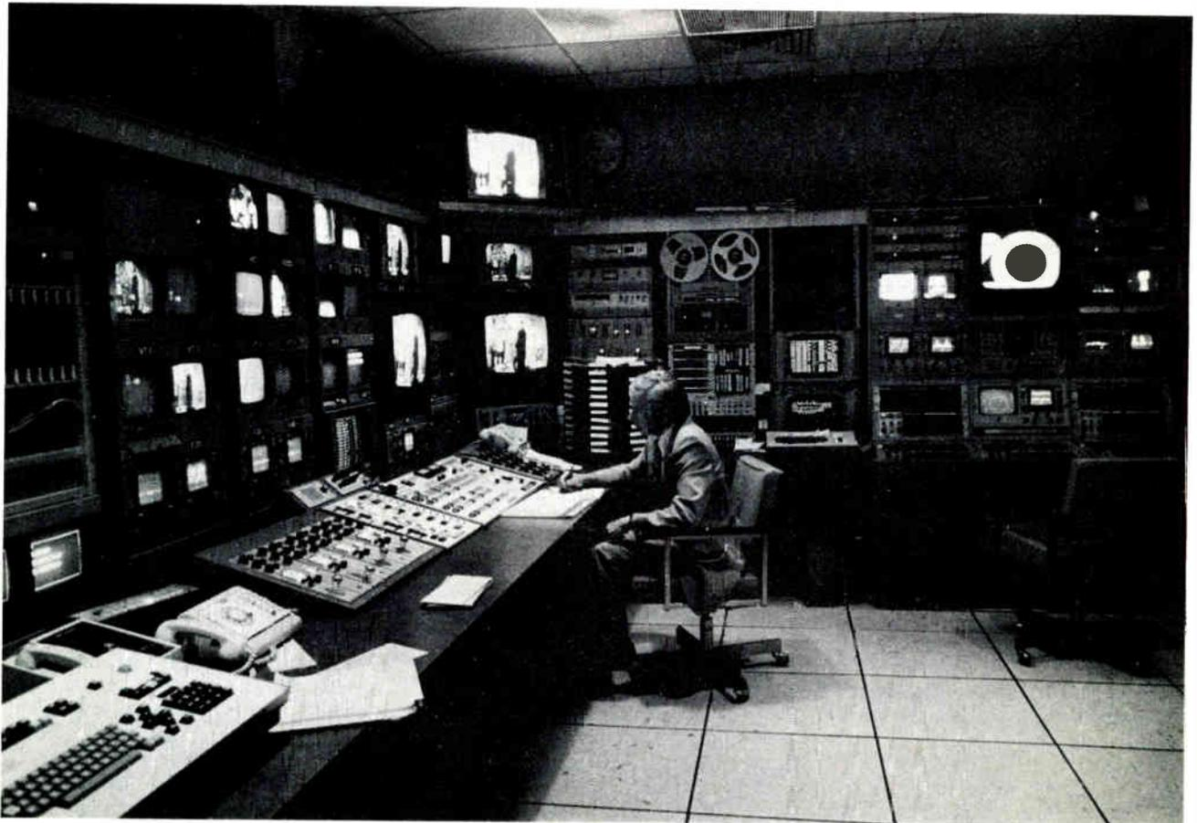
The master control room is supervised by a lone technical director (Larry Johnson) with the air of totally computerized switching system. Program log sequence of upcoming 15 events is observed on CRT terminal directly behind switching console; all events are timed, cut-in, and ended automatically according to preset log.
