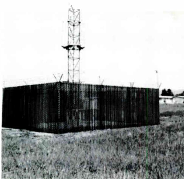
Figure 3 Close-up of tower base shows barbed wire and flood lights included for night meter readings and maintenance.
