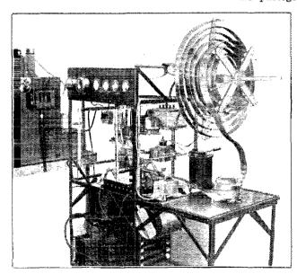
FIG. 10. 11/2-KILOWATT 20-TO 100-METER TEST SET USED FOR OVERLOAD TESTS OF HIGH-VOLTAGE AND HIGH-CURRENT CONDENSERS
