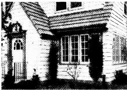
Waterproof concrete tile in color is used here. (Hawthorne Concrete Products Co.)
