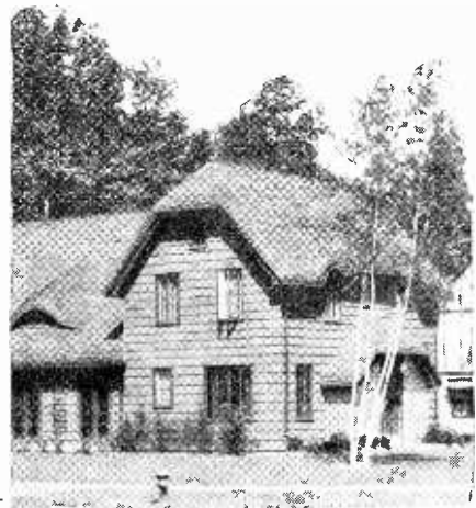
The charm of a thatched roof is gotten with stained cedar shingles. (Weatherbest Stained Shingle Co.)
