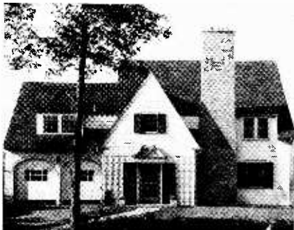
Wood shingles impregnated with preservative stain are moderate in cost. (Creo-Dipl Company.)
