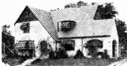
Modern slate shingles of odd dimensions beautify this house. (Penna. Slate Institute.)
