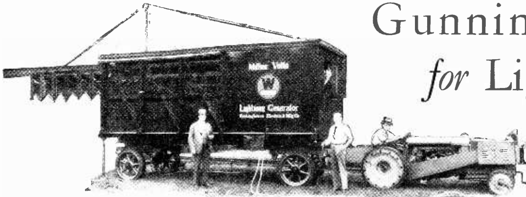
This mobile generator can impress surges of more than 1,000,000 volts on a transmission line.
