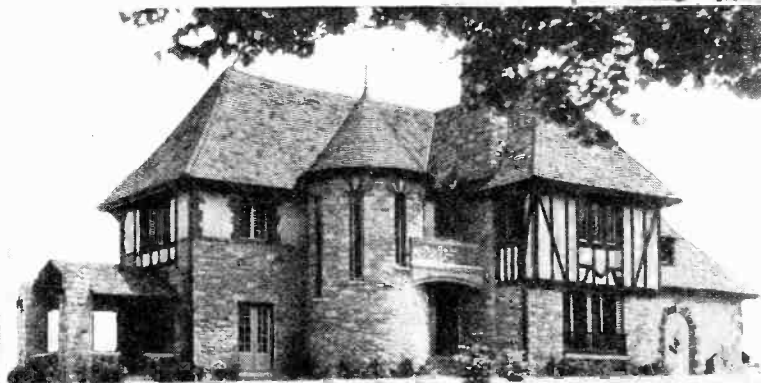
The roof above is of rock-like shale tile. The picture to the right shows how new roofing materials can be applied over the old roof. (Ludowici-Celadon Company; Johns-Manville Company.)
