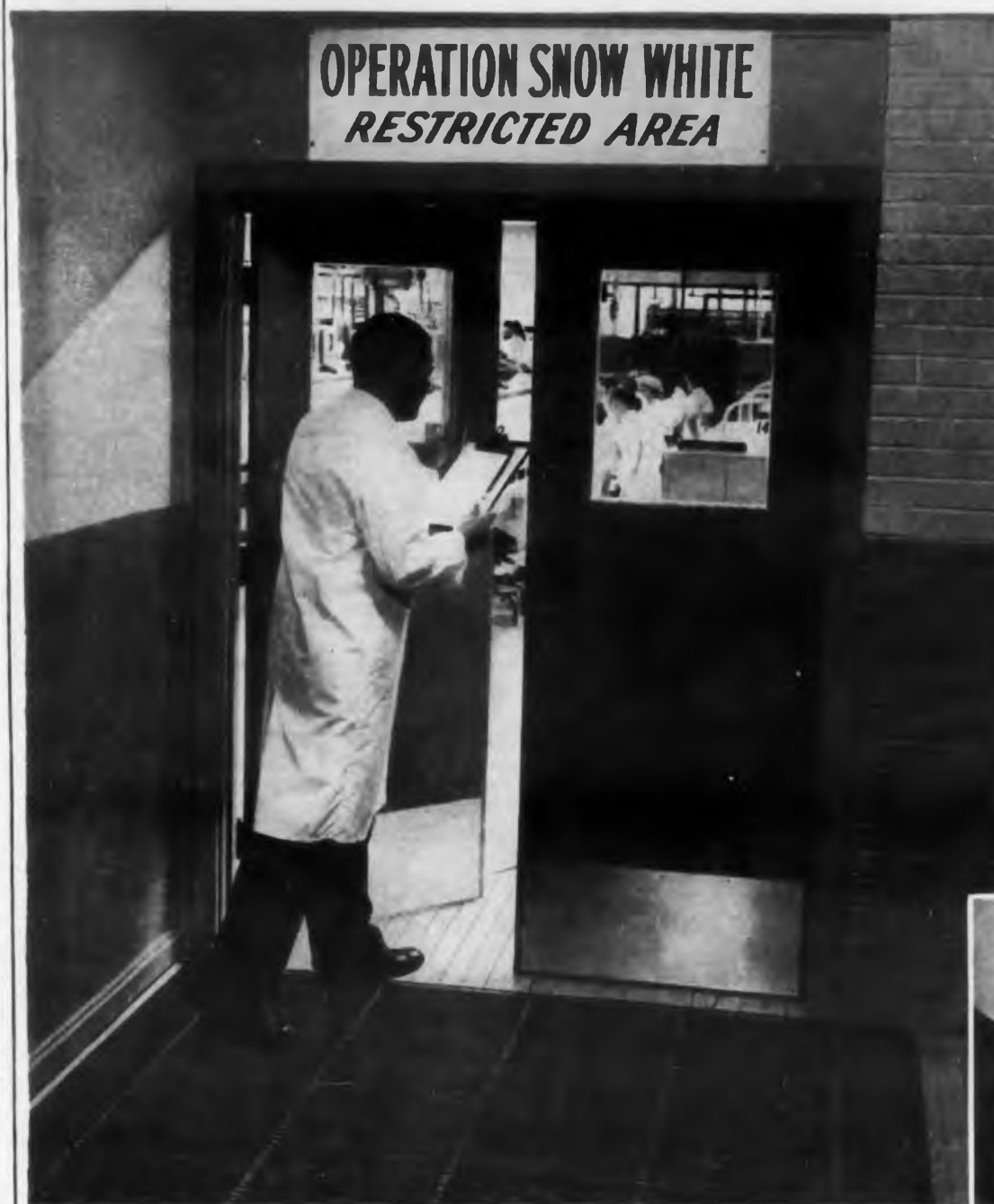
AIR-LOCKS AT ALL DOORS. Employees and other persons entering, pass through air-locks, with a grating underfoot through which powerful suction removes any loose dirt from their shoes. All outer garments, lunches, and personal articles are left outside, in a separate cloak-room. Traffic is closely controlled, and those permitted to enter must wear lint-free clothing. Incoming mail is left in the air-locks, for pick-up and delivery later on by employees who work inside the "Snow White" area.
