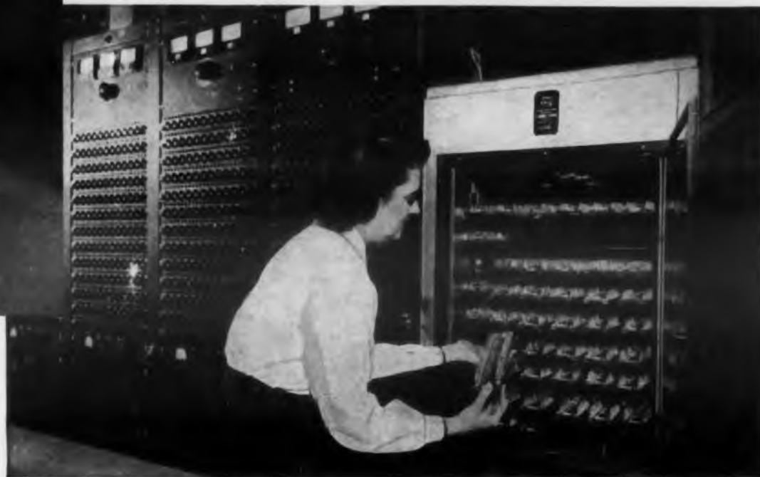
Here rectifiers are automatically tested and inspected in mass quantities.
