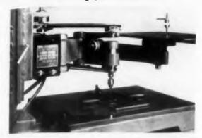
Unskilled operators can drill 100 holes a minute with the model D-2 printed circuit engraver. Various holes can be drilled without changing tools. For two dimensional work, this pantograph has an air cylinder attachment and a single micrometer adjustment for height.
