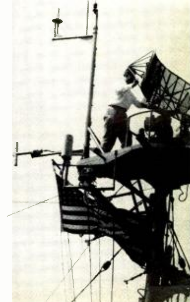
(Left) Adjusting a marine radar to peak performance before installation. (Center) Field engineer boards B-58 to check electronic gear in flight. (Right) Engineers installing a marine radar antenna atop a ship's stub mast.
