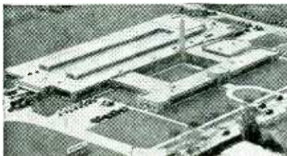
New Sentinel plant in Evanston
