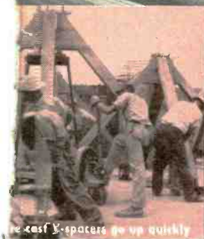
pre-cast Y-spacers go up quickly
