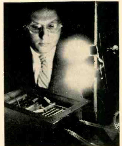
Two 15-watt light bulbs are illuminated by direct conversion of chemical energy to electrical energy by fuel cell
