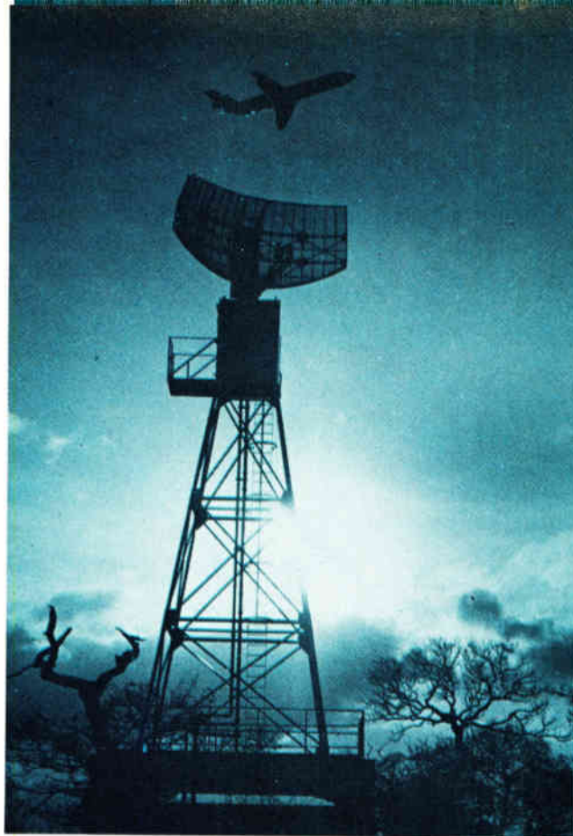
Showing off. Among radars shown at Farnborough was this Plessey S-band model, the AR-15/2, for civil and defense roles.
