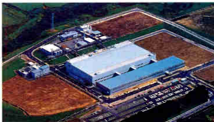
Oki's Miyagi Plant, featuring world-standard process technology and automation.
