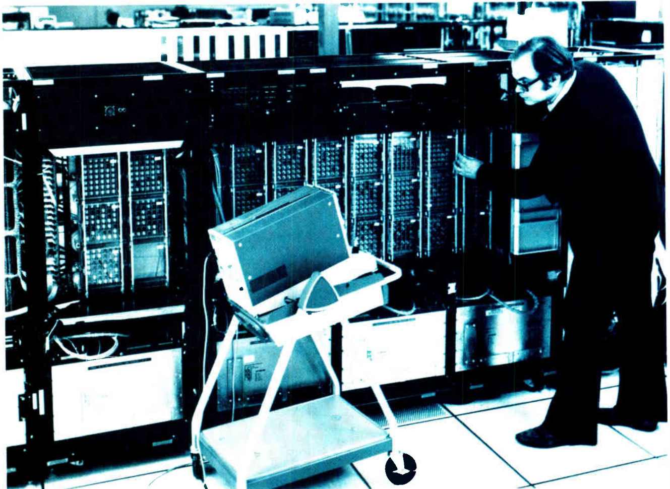
Compatible. Computers relying heavily on LSI, plug-compatible with but much faster than IBM System/370 models, were introduced by companies like Amdahl Corp. Here, the Amdahl 470V/6 gets checked before delivery to the University of Alberta.
