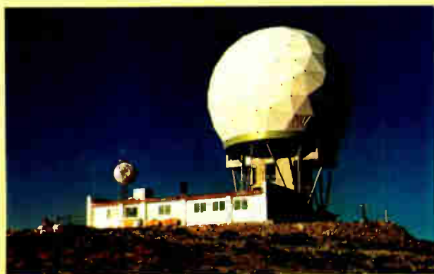
Air traffic control radar station in Mexico, located 3.700 meters above the sea level at CERRO POTOSI - one of the highest radar sites in the world. Connected by a line-of-sight microwave link more than 100 km long to the Monterrey ATC Center.
