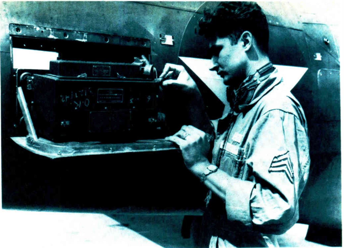
Compact. The war years accelerated developments in radio communication gear, and here too ruggedization and reduction in size became essential, as exemplified by this Army Air Force uhf/vhf command set built by Western Electric, to be installed in fighter aircraft.
