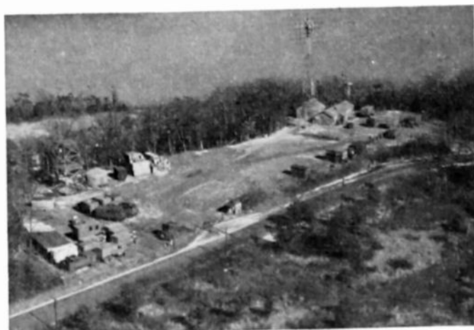
Fig. 8—Aerial view of the moon-radar installation looking in the general direction of moonrise.
