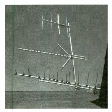
Typical deep fringe installation features VHF-TV Log Periodic antenna at bottom, UHF-TV corner Yagi in middle, and fourelement 2 meter Yagi for amateur VHF-FM at top.
