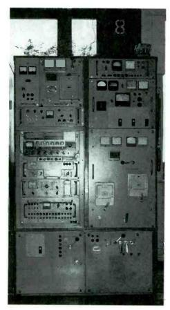
Typical groundwave jamming equipment: communications transmitter "Viaz-M2-OP," 5 kW; 3-30 MHz at Panevezys (Lithuania) site. (Photo by Rimantas Pleikys)
