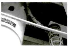
A length of Radiax winds its way through the underground complex all the way to the bottom of the silo. Without the Radiax, communications from the control center to crews elsewhere underground would be impossible because of the extensive shielding.
