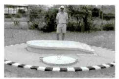
A museum guide (for scale) stands near one of two IRCS backup antennas in the "stowed" position. These can be fully deployed in about 50 seconds. The foreground hatch is a service manhole.
