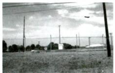
Figure 1. NXX/388 kHz, Willow Grove, PA – Transmitter is housed in the small shed; antenna wire is strung between the utility poles.
