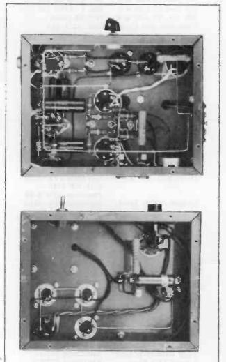
Figure 6. Bottom Chassis - Stancor-Williamson Amp.
