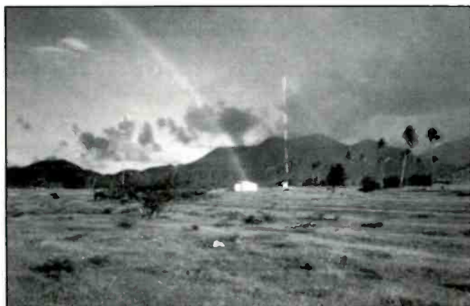
The "new" Caribbean Radio Lighthouse 1160 kHz transmitter site.
