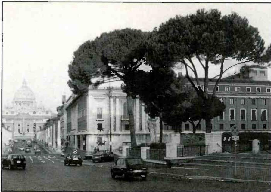
This building houses the production facilities of Vatican Radio.
