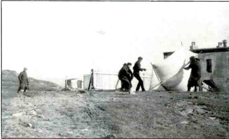
Marconi watches at a distance as his staff struggles with the kite that was needed to lift the receiving antenna.
