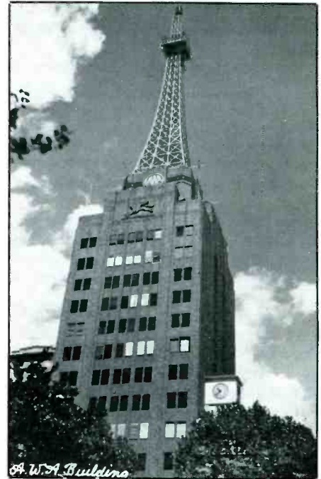
That's not the Eiffel Tower on top of this building. It's the antenna of station 2CH, Sydney, NSW, Australia. (Courtesy Hank Milten, IA.)
