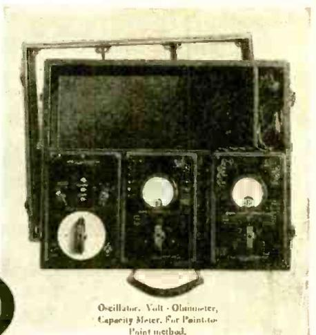
Oscillator, Volt-Ohmmeter, Capacity Meter. For Point-to-Point method.
