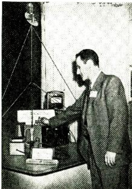
Photo E—The G-string u.h.f. antenna.
