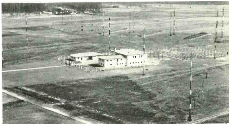
Radio Free Europe operates this transmitting station in Biblis, Germany.
