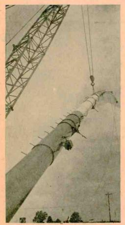
pole was assembled and painted, and the aircraft warning lights installed and wired. The three lower sections had the wire rope slings in place with the come-a-longs (coffin hoists) in tension. Before raising the pole into position, a tag line was fastened at the top of the pole and another one about half-way down. Taking care to protect the aircraft warning light at the top of the pole, workers fastened the wire sling at the balance point of the pole.
