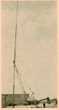
Coop engineer Wiley Jones (sweater) checks pole position over anchor bolts before pole is lowered into final position. Once pole had been seated on anchor bolts, workmen then adjusted first leveling nuts, then anchor nuts to ensure that entire 247-ft-high structure was both adequately secure and accurately locked in true 90-degree-from-horizontal position.
