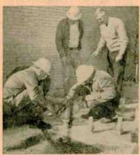
Below, left, ten 80-in. anchor rods made up pole's anchorage. Below, right, Alois Luhr (no hat) checks pole's 16-ft-deep foundation.
