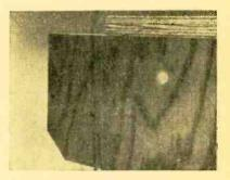
About 1-in. of bottom rear corner of vertical supports should be mitered off to allow space far line cords and other wiring to pass along table top between platform and wall. Supports should extend about 3 in. beyond top of platform at rear to prevent equipment from being pushed flush against wall.
