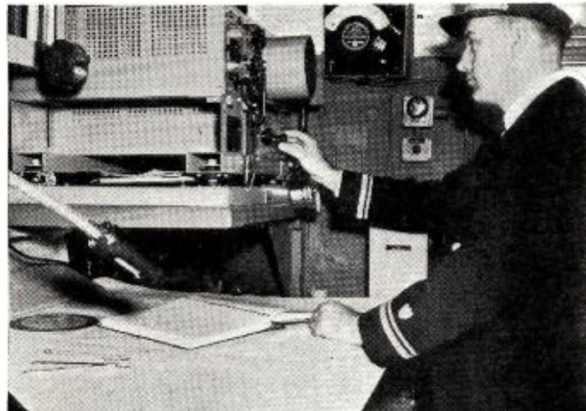
Fig. 4. Loran receiver indicator aboard a Coast Guard vessel.
