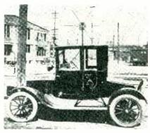
In 1927, the Portland (Ore.) Electric Power Co, used this radio-equipped auto to trace down interference with radio reception in the locality. Believe it or not, equipment in the coupe could be used to find the exact location of disturbing noises.
